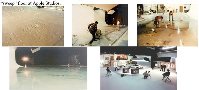
The requirement was to get a smoothness (flatness) such that a Kleg light at ankle height in a dark room wouldn't cast a shadow. I estimated that this would be an Ff of 200+ or so. It took 2+ weeks of work with successive grinding and patching to achieve this, just in time for an Easter photographic shoot with their major customer. This is a \$30-\$50/sqft repair today.
