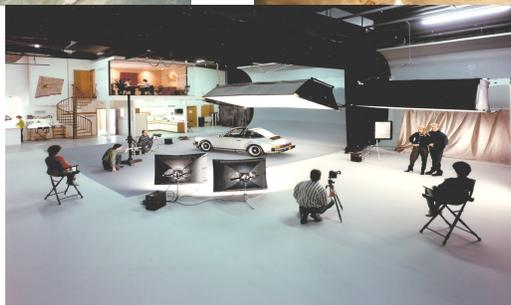
The requirement was to get a smoothness ( flatness) such that a Kleg light at ankle height in a dark room wouldn't cast a shadow. I estimated that this would be an Ff of 200+ or so. It took 2+ weeks of work with successive grinding and patching to achieve this, just in time for an Easter photographic shoot with their major customer. This is a \$30-\$50/sqft repair today.
