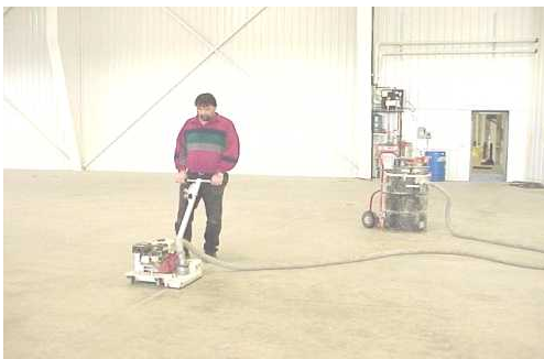
SAW CUTTING JOINT WITH VACUUM
