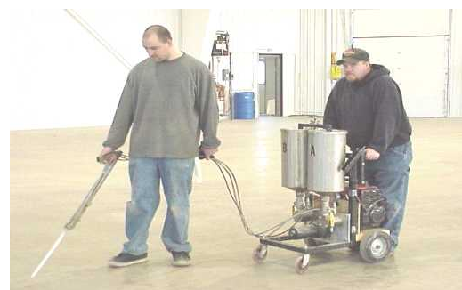
FILLING JOINT WITH PFAC
