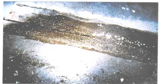
FILLING JOINT WITH PFAC
