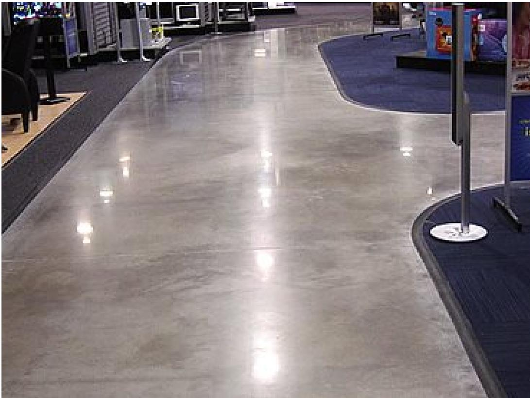
At a level 3 polish, your concrete floors will really begin to shine and clearly reflect side and overhead lighting.
