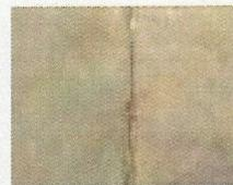
Unfilled joints will spall and deteriorate under heavy wheeled traffic.
